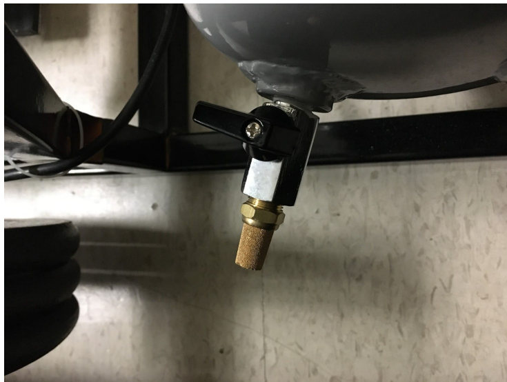
Figure 28A. Close up picture of manual draining valve.
